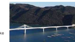
"Bizen Hinase Bridge" in Okayama
