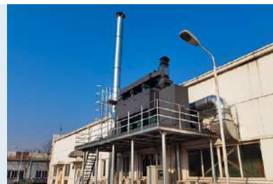
Combustion vulcanization gas treatment equipment Tokai Rubber Moldings (Tianjin) Co., Ltd. (China)
