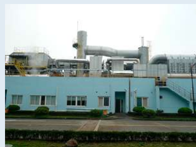
Combustion type VOC processing equipment Tokai Rubber (Jiaxing) Co., Ltd. (China)
