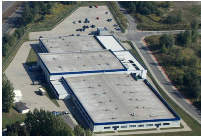
Expected site of the SRK-HP plant to being operation in the fall
